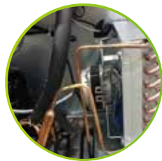
Defrosting Water Self-evaporation Design, No need drainage
